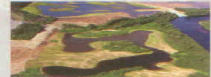
Wetland created in a borrow pit (Péribonka hydroelectric development)
